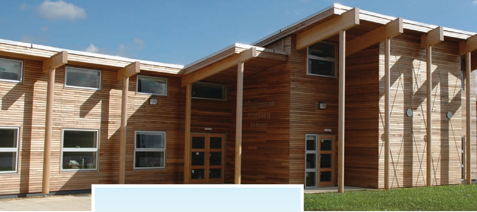
ABOVE: The main structural element of the school is a large glulam-inated frame of timber from a sustainable source. RIGHT: The classrooms are naturally ventilated through windows and rooflights. FAR RIGHT: Natural lighting is maximised in the north-facing classrooms
