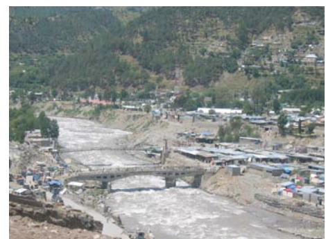
Fig 10: Bridge over Kunhar River under repair, Balakot.
