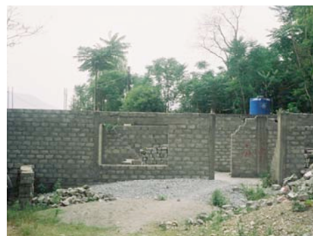
Fig 33: Infill masonry finished on ground floor, Balakot.
