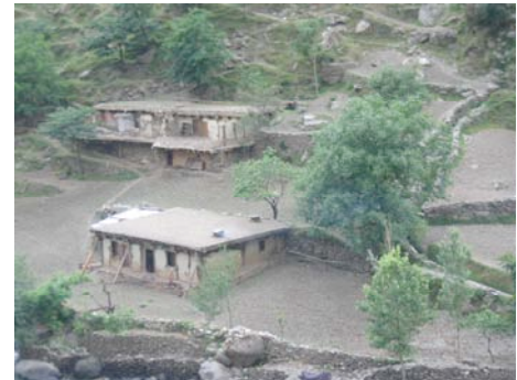
Fig 27: Stone and timber house in Khaghan Valley. Propped but still standing .
