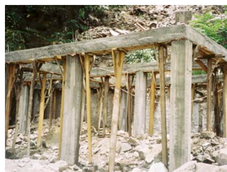
Fig 31: Concrete frame under construction, Balakot.
