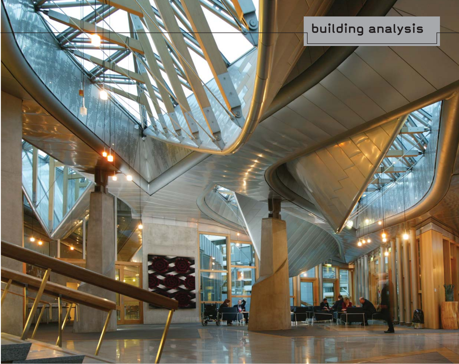
ABOVE: The garden lobby is one of several parts of the building that uses natural ventilation
