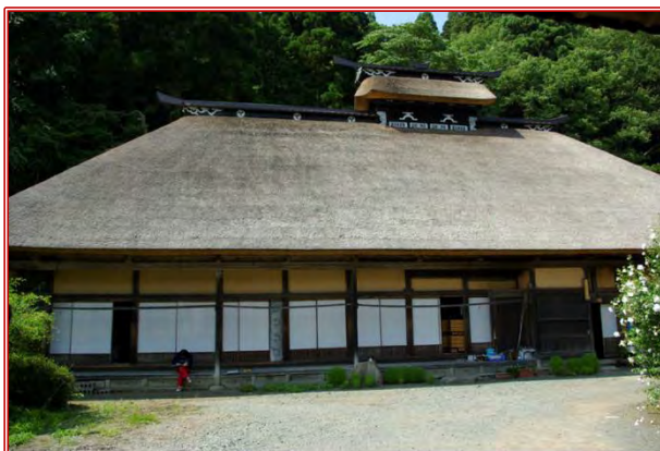
Figure 6.10 (Left) Ogata House before the tsunami.
