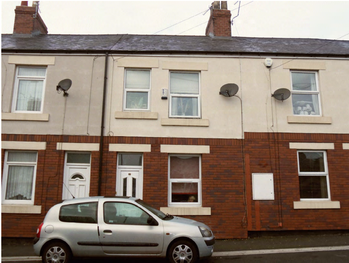
External insulation in impermeable render and brick slips, Stockton. Unintended consequence: condensation.
