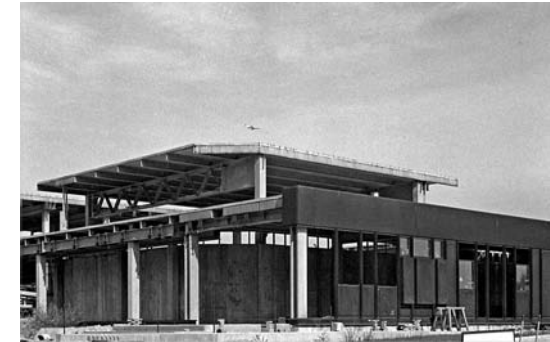
Figure 1 The Free University, Berlin, under construction in 1970 (Candilis Josic Woods, architects). A complicated kit-of-parts construction system provided opportunities for reconfiguration that were never used.
