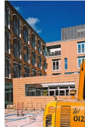
Figure 6. The sizing of seminar rooms in the new Faculty of English building in the University of Cambridge (Allies and Morrison, architects, 2004 – above) was based on an approximation to the positive Poisson distribution, to provide flexibility when there is uncertainty about the size of seminar groups.
