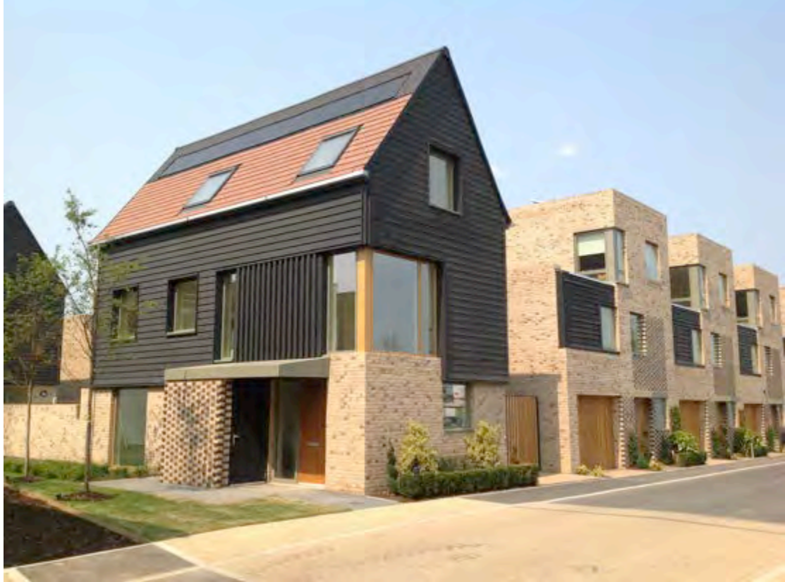
Abode, Great Kneighton, Countryside Properties. Proctor & Matthews Architects. Civic Trust National Panel Special Award 2015.
