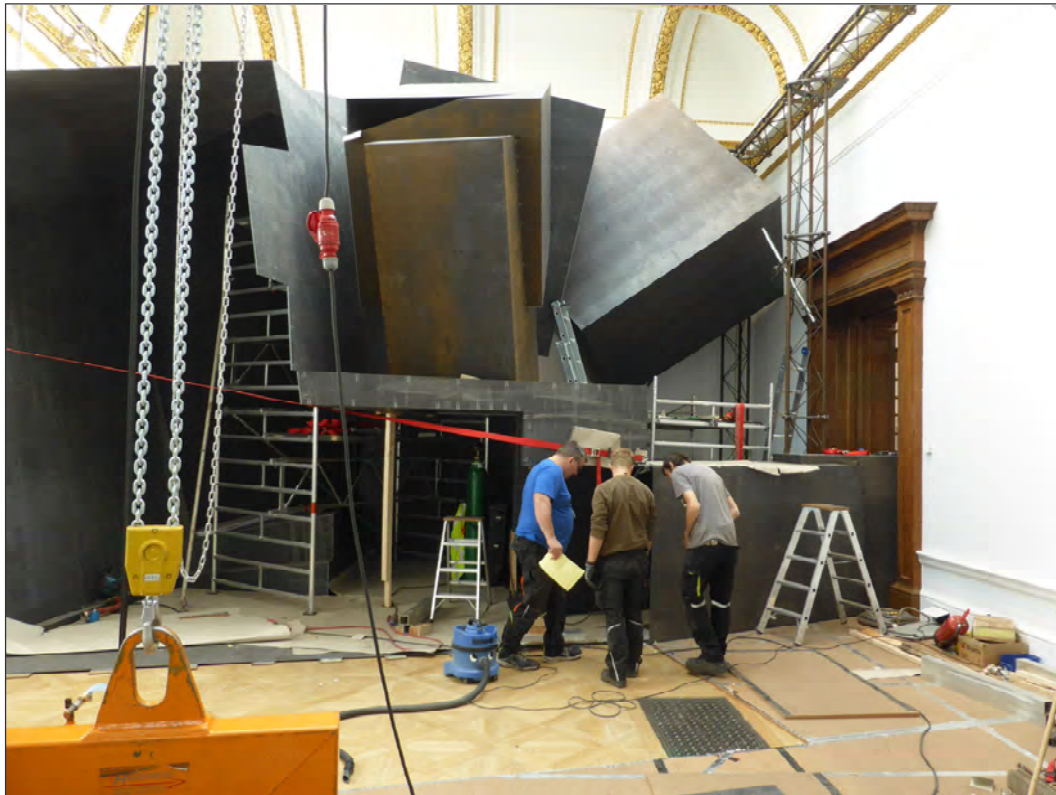
The RA was a construction site for 3 weeks before opening day
