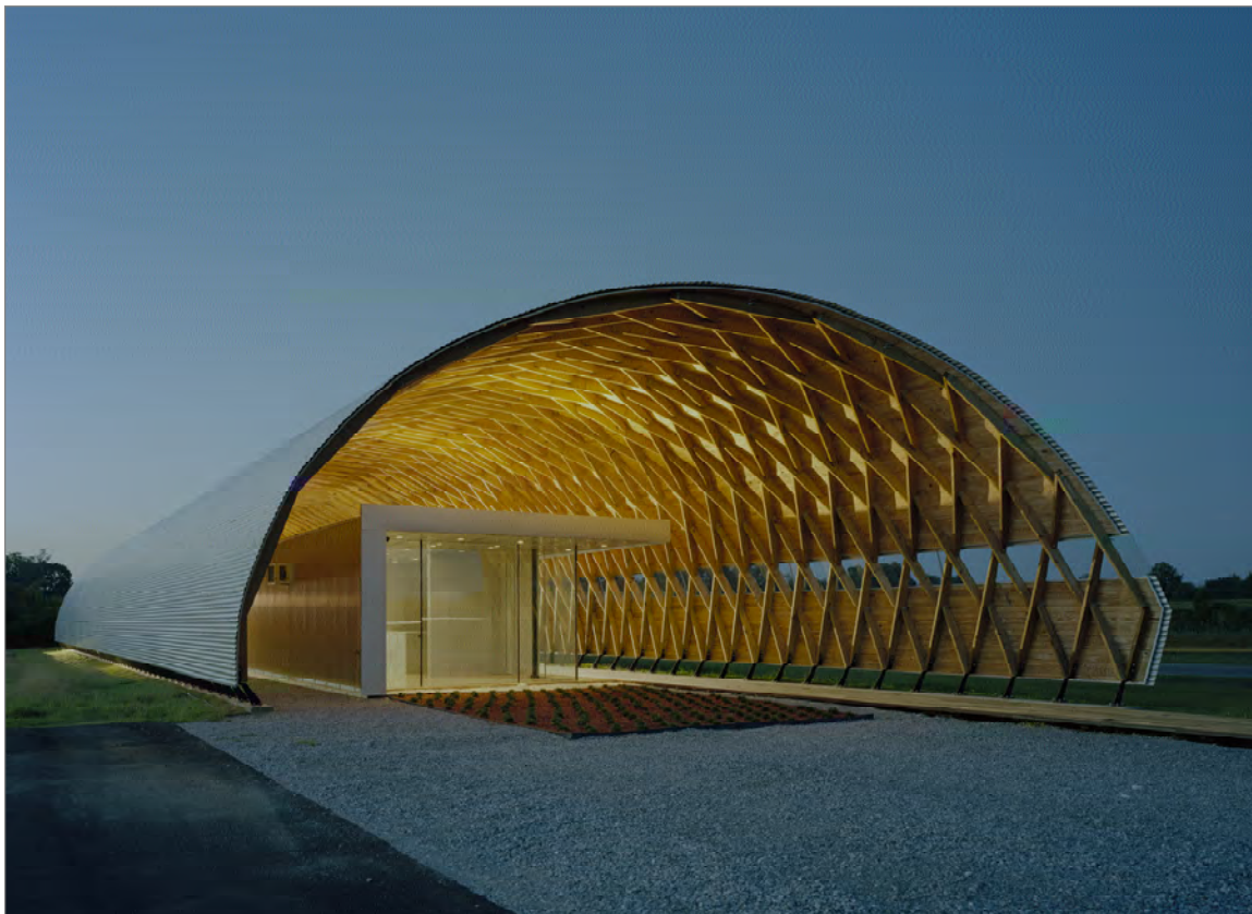
Greensboro Animal Shelter, Alabama A lamella barrel vault structure realised by Rural Studio Thesis Students 2012
